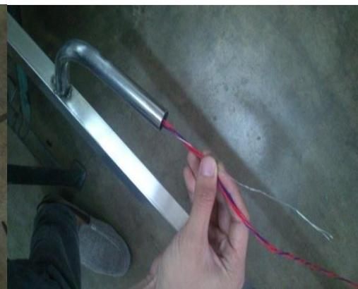
**6. Install the wire for the sensor and for the siren. Wires should be inside the boom and must be connected tightly using the soldering iron**
