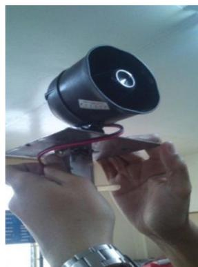
**7. Install the siren to the siren holder. Proper wiring should be done to make the siren functional during emergency**
